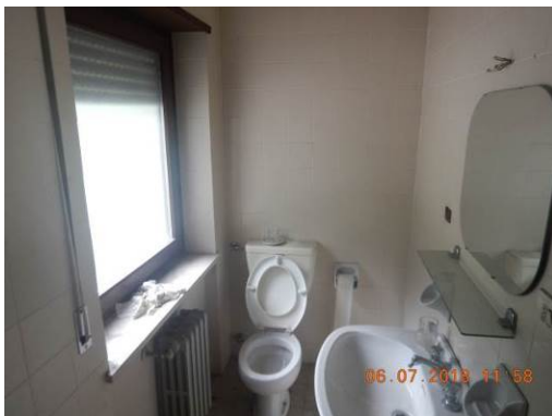
Bagno 1 – Piano terra
