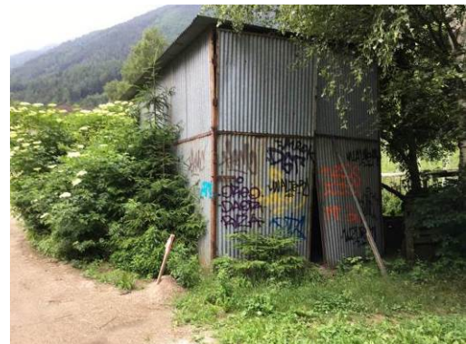
Baracca – Barackenlager “A8”
